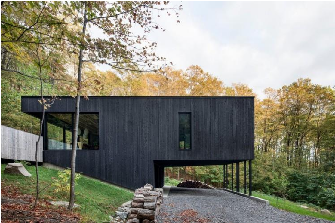
Figure 3.1 – A precedent showing how a building can be constructed using a pilotis construction method to work with site level changes. We believe something similar to this will be produced underneath the main body of the building to which we will submit full details of to the full satisfaction of the local authority.
